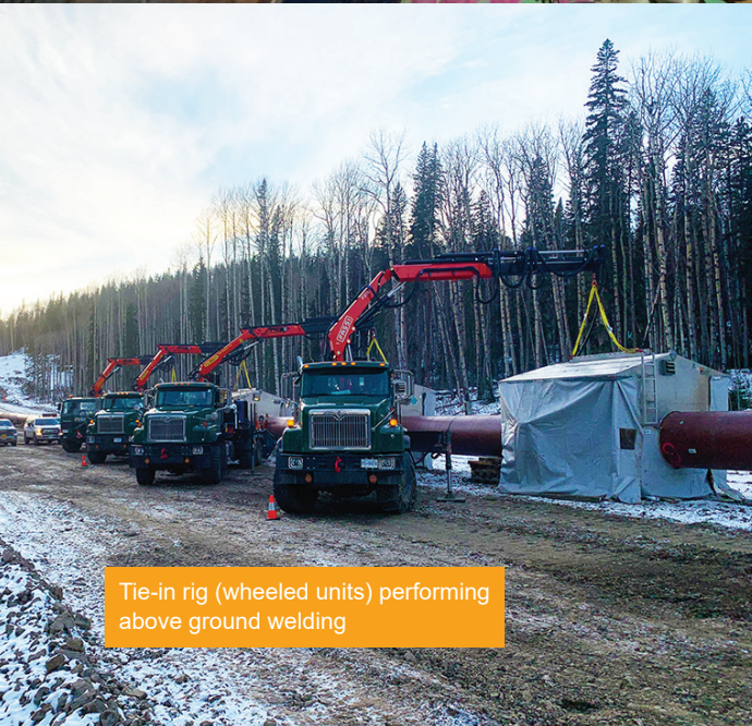
M300 in progress
